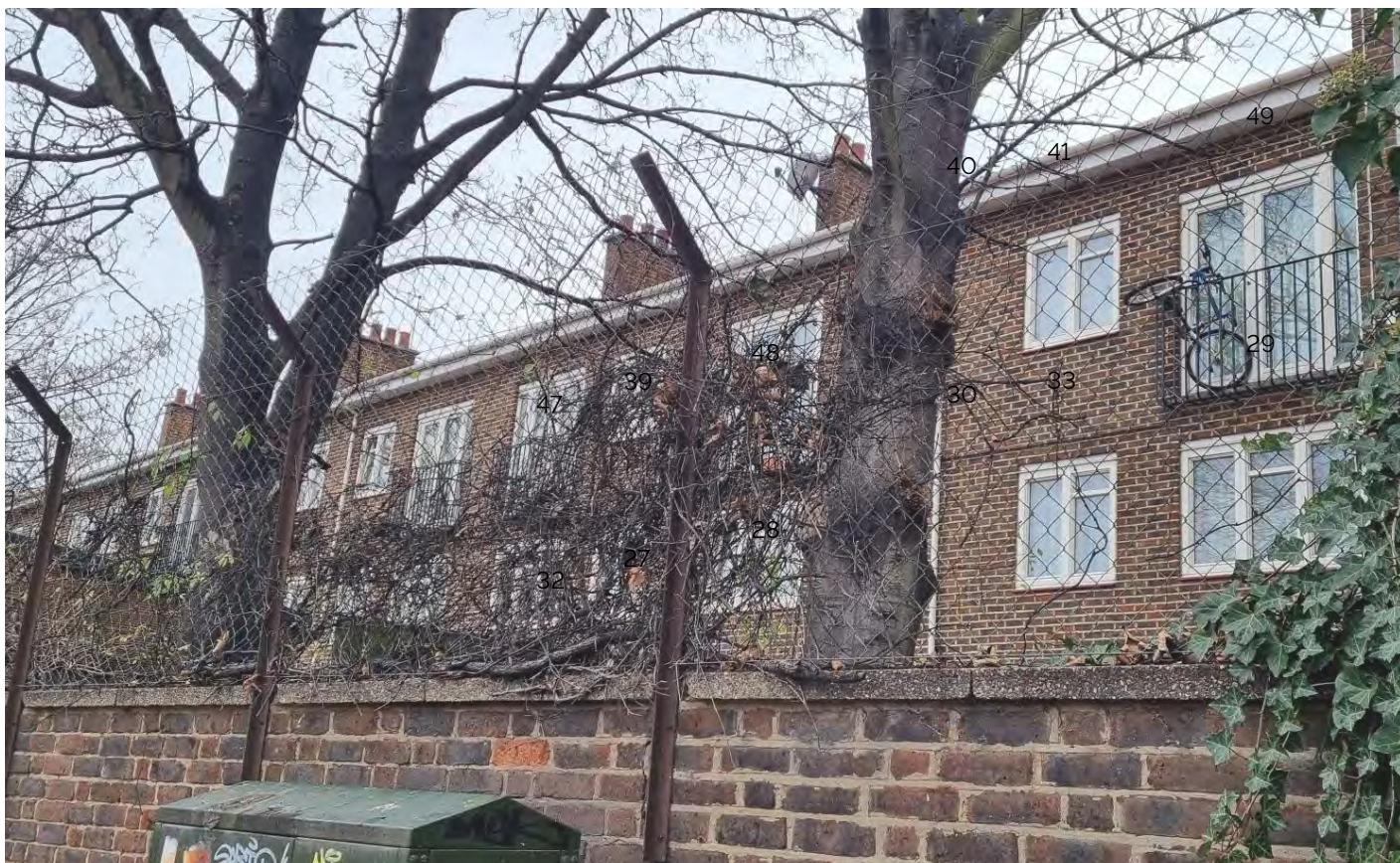
Figure 2. Window numbers - 1-29 St Matthew's House
