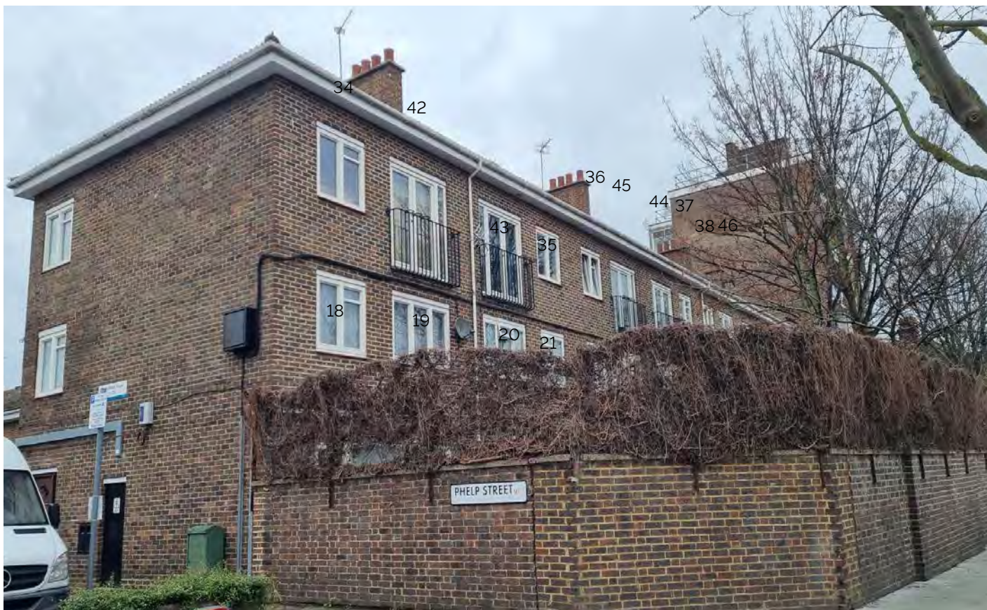
Figure 1. Window numbers - 1-29 St Matthew's House
